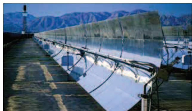
Solar-thermal parabolic trough power plant
